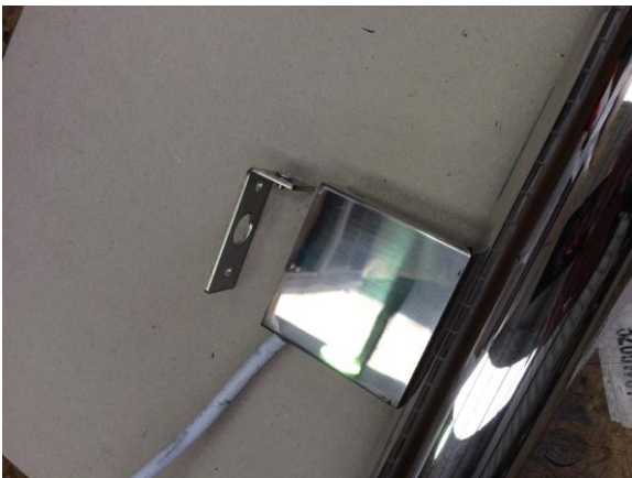
Fig 1 Exposed wiring
